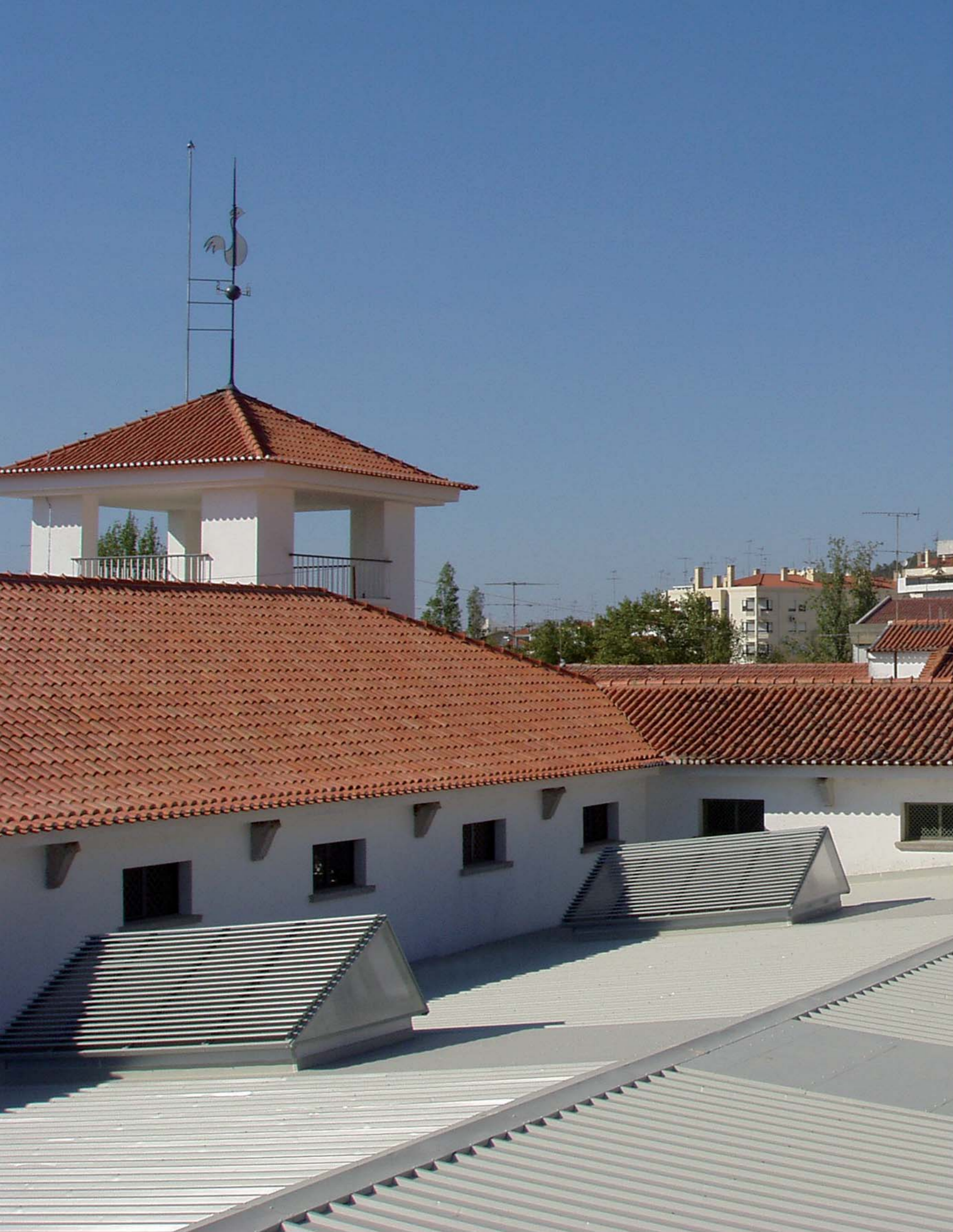
Illustration: Asymmetrical DELTALIGHT with solar shading on the side facing the sun.
