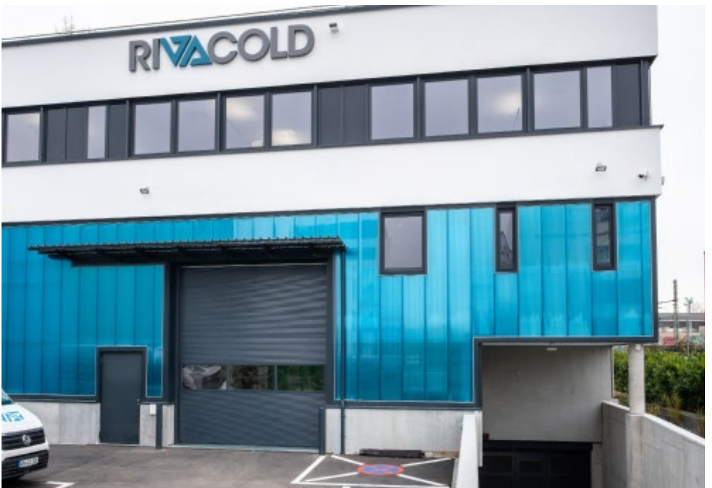
Unique building facade with over 250 square meters of lighting elements
