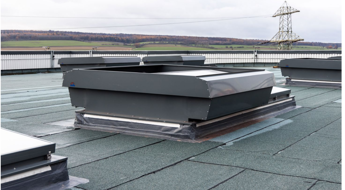
Multi-purpose ventilator type MEGAPHÖNIX for air exchange independent of weather conditions.
