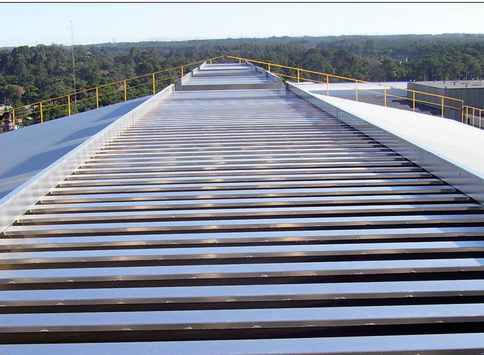
Large illustration: AIRSTAR labyrinth ventilator spread along the whole ridge of a factory building.
