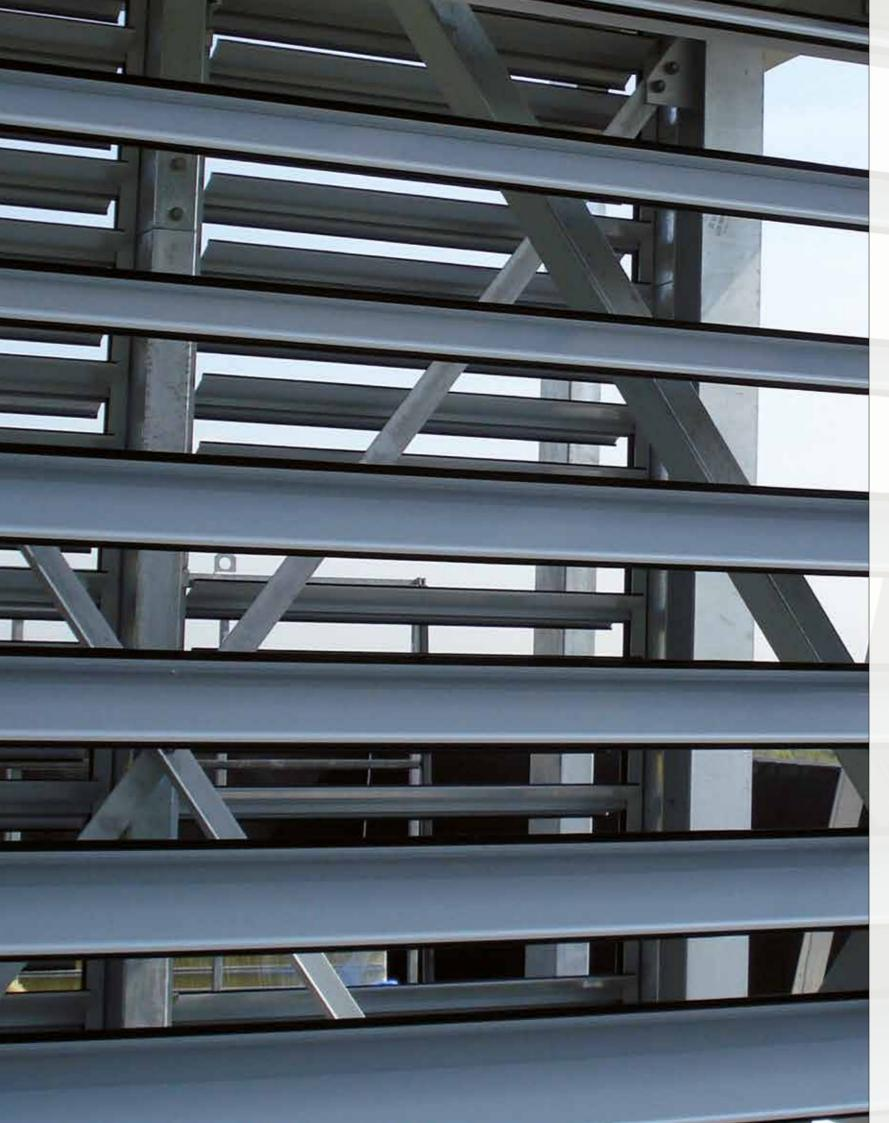
S 200 The S 200 is an economical solution for industrial use as a supply air system, which is also designed to serve as a shading or privacy screening system. The frame is made of extruded aluminium profiles with a frame construction depth of 50 mm and a frame face width of 38 mm. The S200 is approved as a smoke and heat extraction system according to DIN EN 12101-2:2003. Louvre blades:
